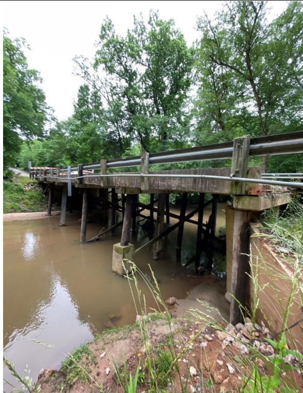
Photograph 4 – S-294 Bridge Facing South
