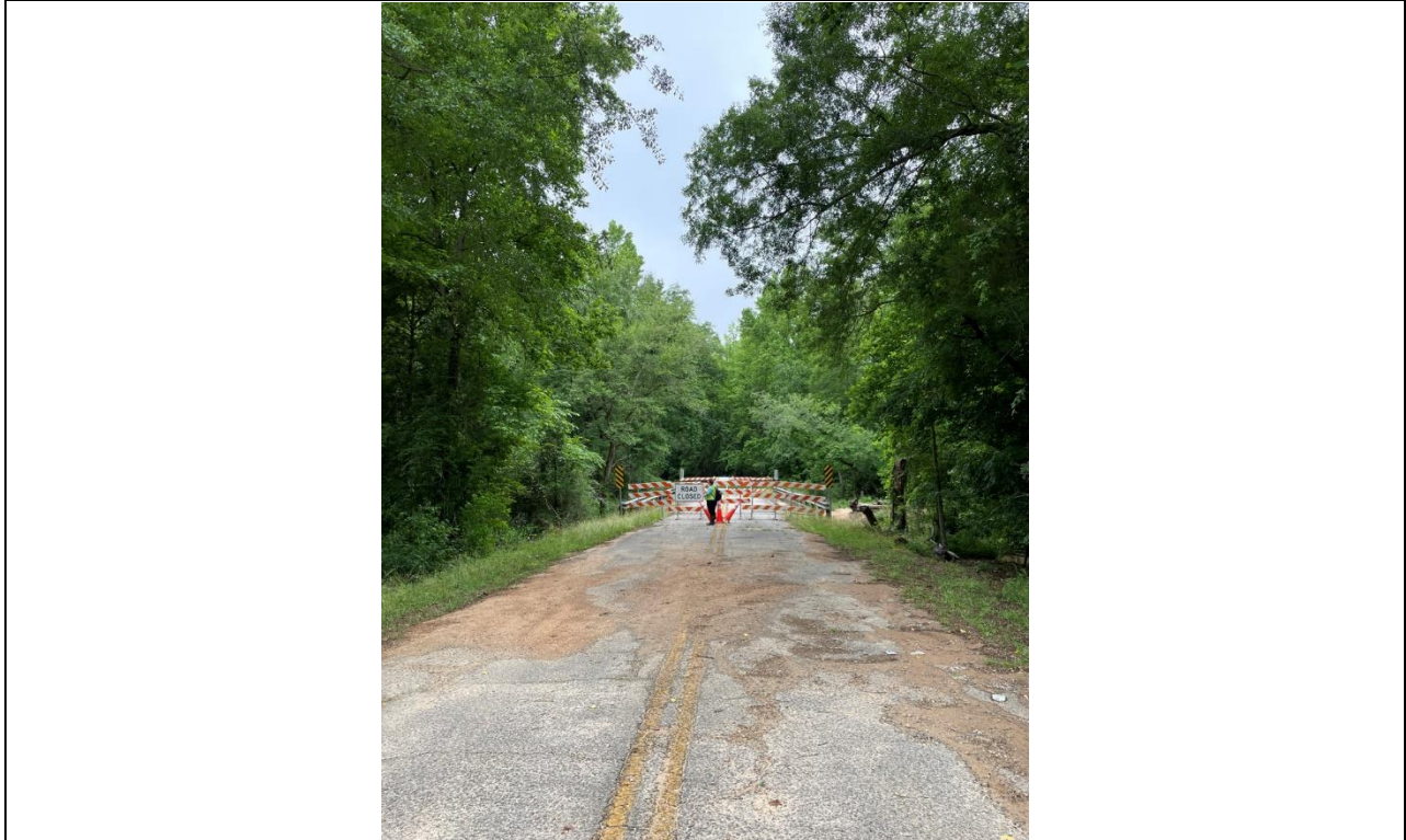
Photograph 1 – S-294 Bridge Facing West
