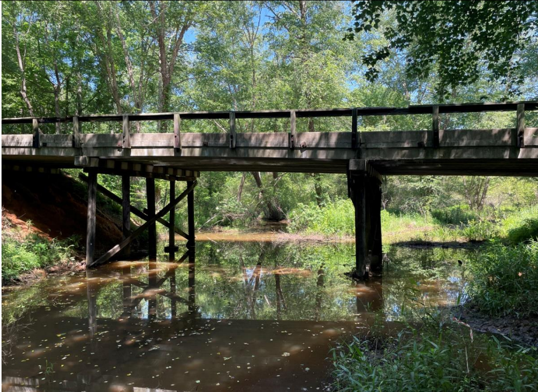
Photograph 7 – Stream 1 (Hanging Rock Creek) Facing West
