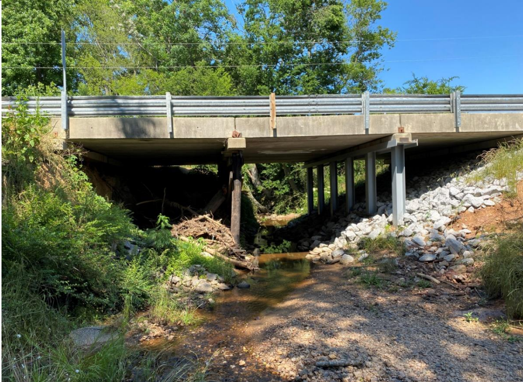
Photograph 4 – S-108 Bridge Facing East
